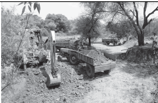
Silt removal in Eguvabai Kunta during April 2013
