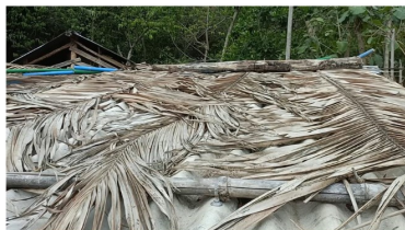
Insulation of shed with palm leaves
